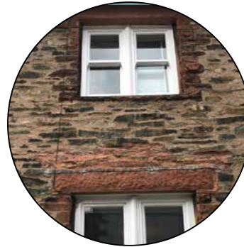
Red sandstone window surrounds and window headers.
