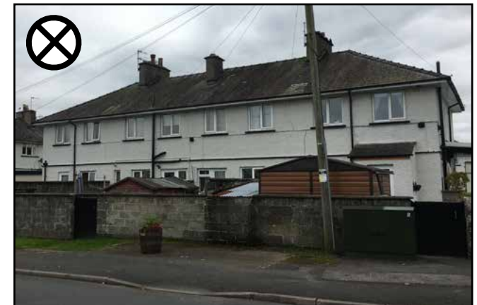
Figure 85: A lack of screening reduces privacy. Breezeblocks are an unattractive boundary treatment
