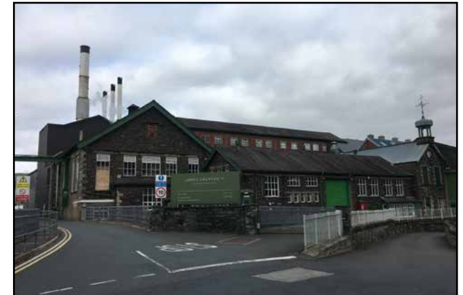
Figure 48: The paper mill and its chimneys form an important industrial legacy
