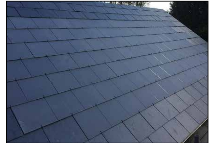
Figure 105: Solar panels can be adopted to look like original slate roofing
