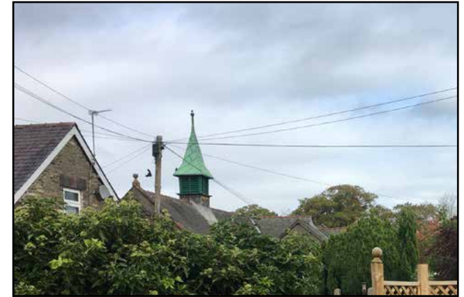
Figure 59: Views of the village hall spire
