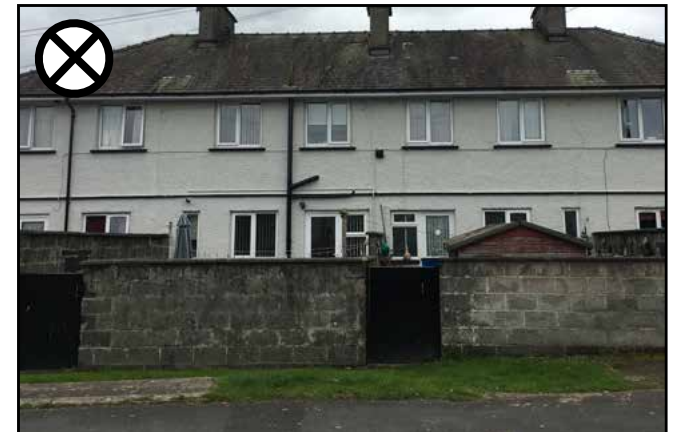
Figure 94: Breezeblocks do not age well and are considered inappropriate
