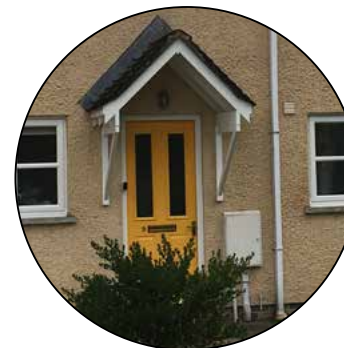
Pitched roof porch.
