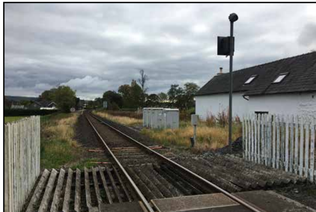
Figure 28: Views south along the railway line
