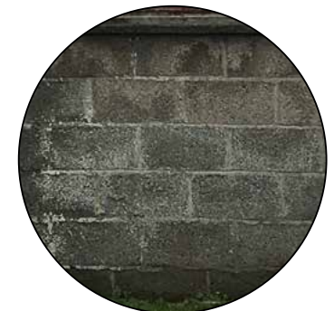
Exposed breezeblock should be avoided.
