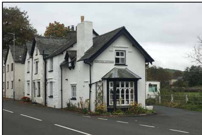
Figure 33: Grade II listed Junction Cottages
