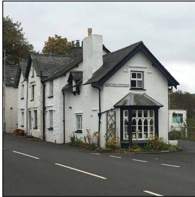
Photograph 5: Junction Cottages, Burnside Road
