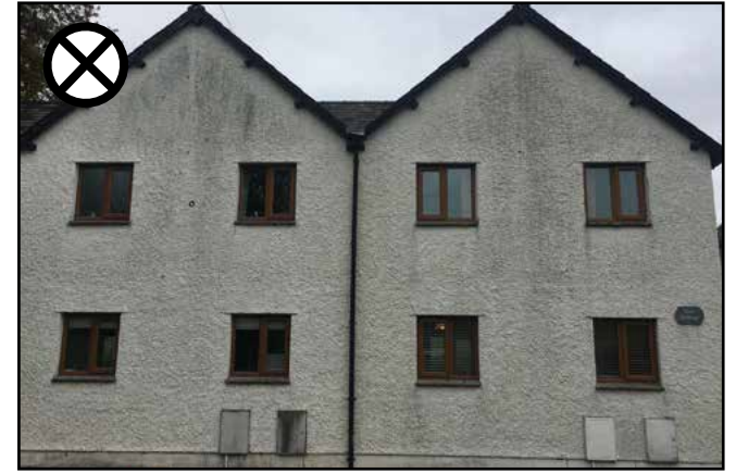
Figure 103: A lack of detailing and an uncharacteristic solid to void ratio for the area
