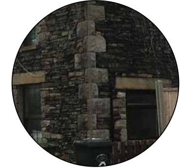
Traditional stone quoins against limestone.
