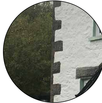
Stone quoins against a white painted facade.
