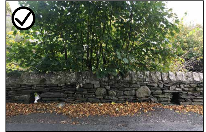
Figure 54: Drainage features accommodated within traditional stone wall
