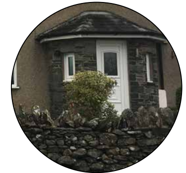
Stone porch with a hipped roof.
