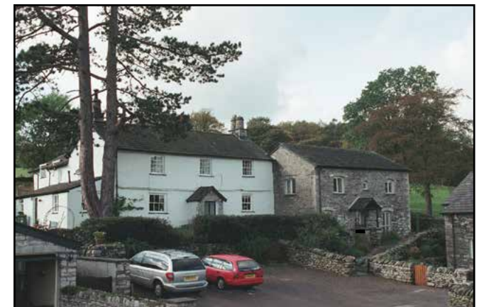
Figure 34: Grade II listed Hollins Farm
