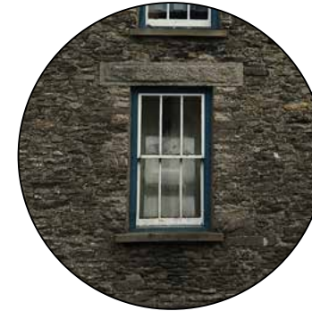
Retaining the original window sub-division is encouraged.
